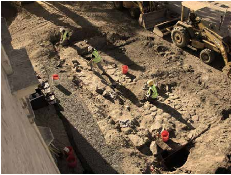
Figure 17. View of the archaeologically-exposed granite foundation footings, boulder pavements, and Roman mortar floorings of the Serra Chapel of 1772. The archaeology field crew, consisting of Gerald Jones, Esther Kenner, and Brenna Wheelis, respectively, are here pictured recovering the granite-boulder pavement of the Serra Chapel of 1772; the footprint of which is located within the forecourt of the San Carlos Cathedral. Photo © Rubén G. Mendoza, 2008.
