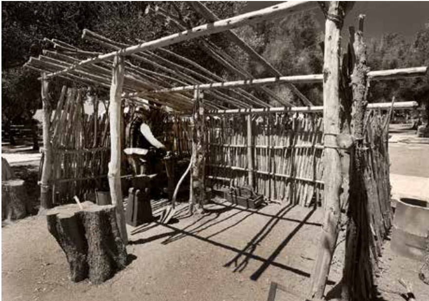
Figure 13. The construction of a jacalon or pole-and-thatch structure was recently undertaken as part of an ongoing restoration and public education effort by the Mission Conservation Program of San Juan Bautista. The structure in question provides an approximation of what one might imagine for some of the earliest structures once located at the Royal Presidio of Monterey. In this instance, construction required the preparation of rawhide straps for use as ties for binding together those poles forming both the perimeter walls and roof of the structure. The effort was directed by program docent and blacksmith John Grafton with the assistance of a host of CSU Monterey Bay student interns. Photo © Rubén G. Mendoza, 2013.
